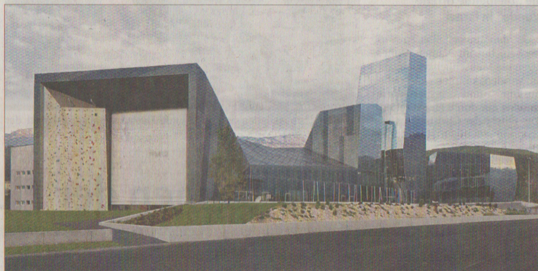
Salewa Headquarters in Bozen-Süd
